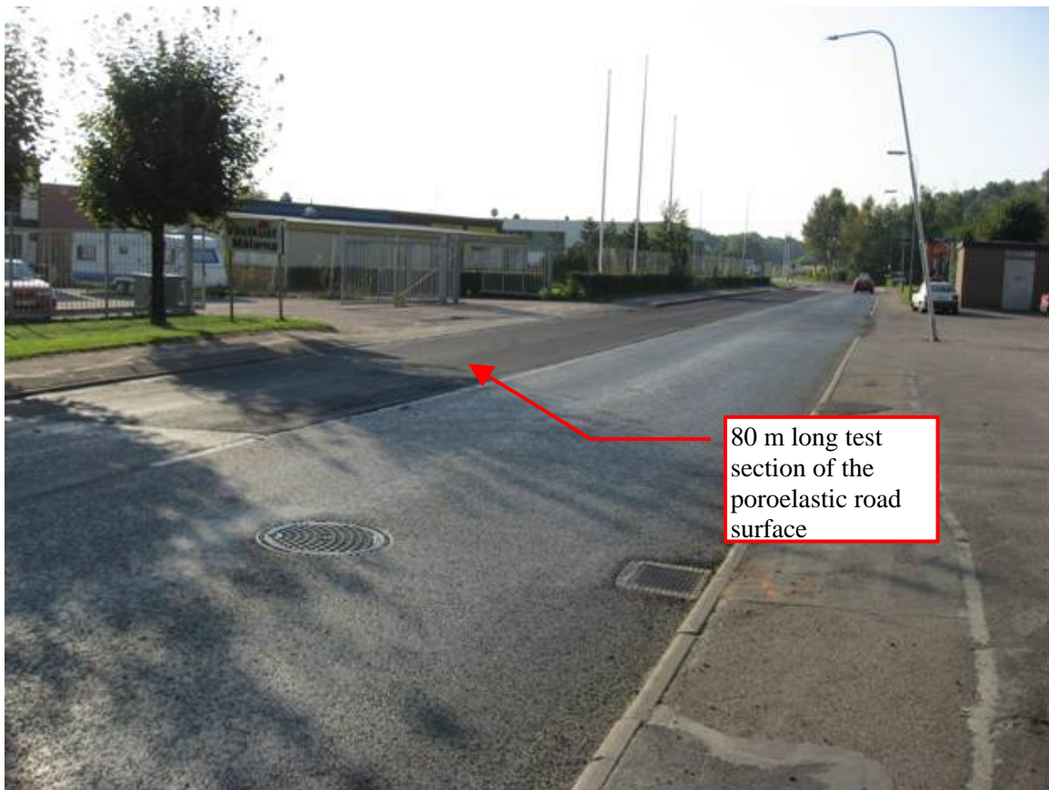
Figure 9. The poroelastic road test section at Tagenevägen in Göteborg.
